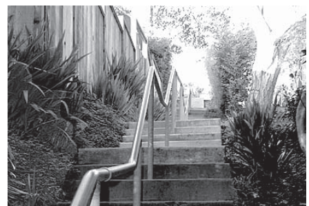
Martinez Path - new handrails and repaired steps improve safety
