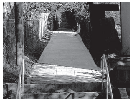
Easter Way - repairs of cracks and tilting improve walking
