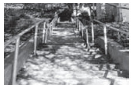
Billie Jean Walk - new handrails improve safety on steep steps
