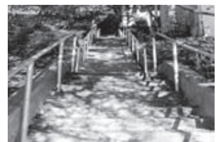
Billie Jean Walk - new handrails improve safety on steep steps
