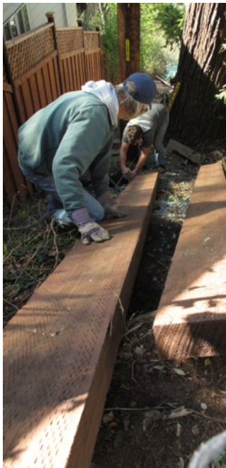
Installing stairs on an especially steep section of path
