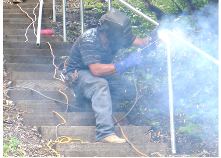
Installing the handrails on La Loma Path
