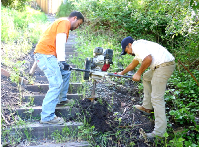
Installing the handrails on La Loma Path
