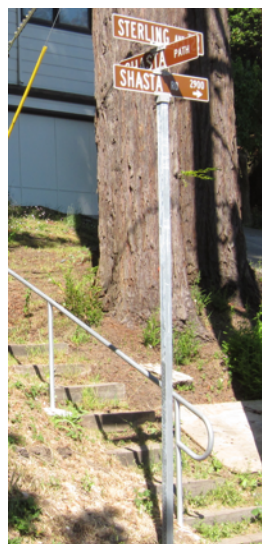
New handrail at the bottom of Shasta Path
